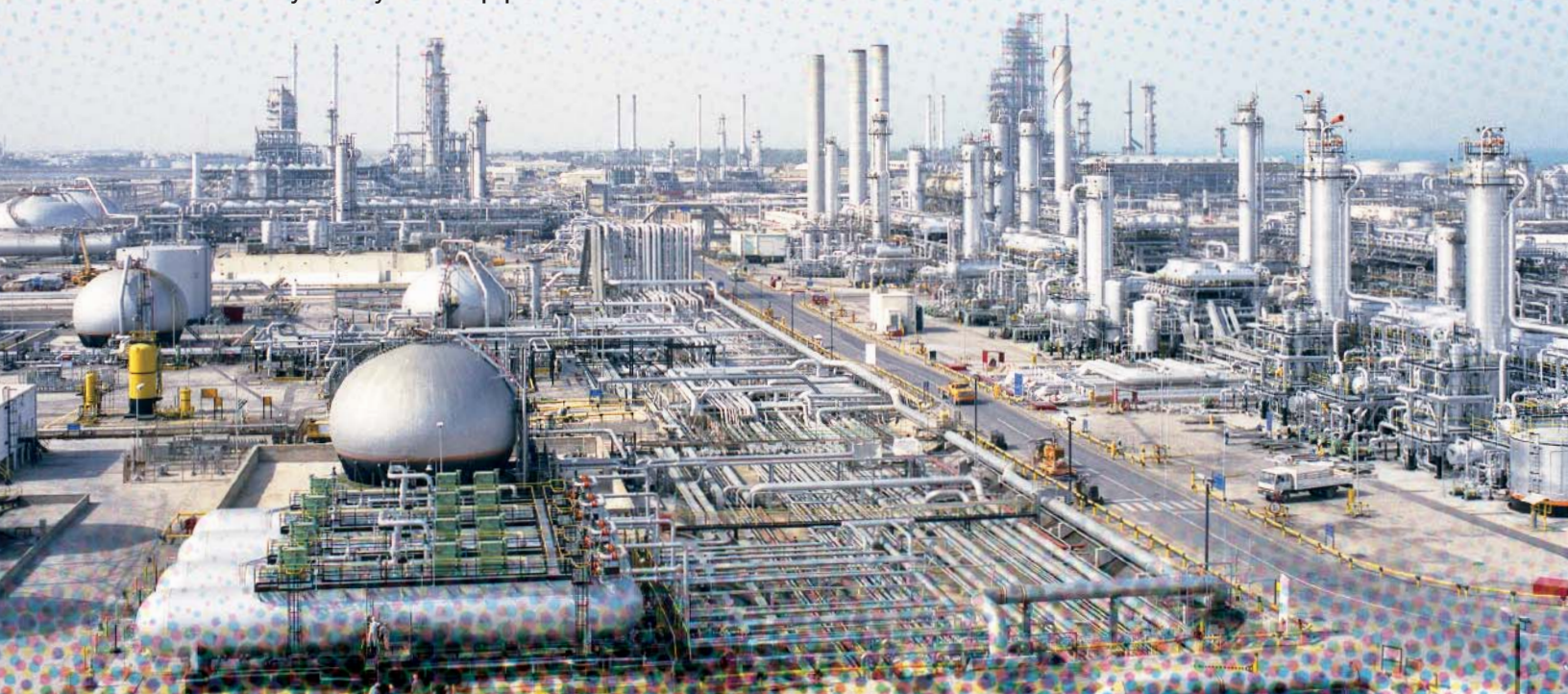
Ras Tanura Refinery’s key executives, at top, are Ibrahim K. Al-Naimi, left, manager of the Refinery Operations Department, and Abdullah S. Zaindin, manager of the Refinery Maintenance Department. Below: The refinery is a labyrinth of equipment and facilities.
